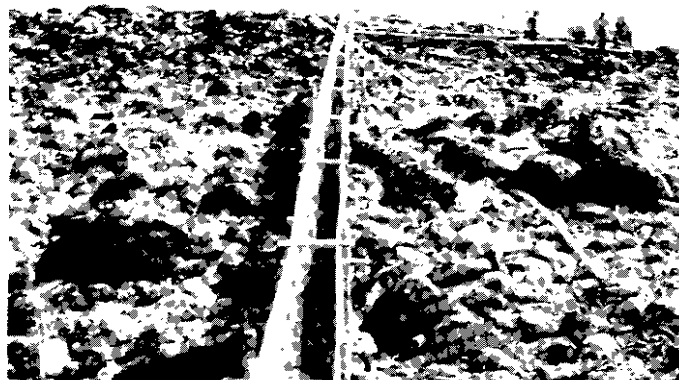
Placer Training Camp, Fraser River at Mouth of Emory Creek near Yale. Main Sluice and Laterals.
