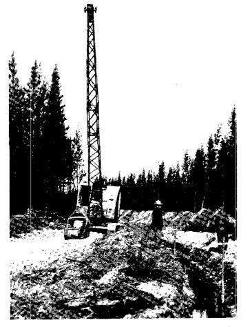
Ditch-construction using boom drag-line, Germansen River, operation of Venture Exploration Co. (East Africa), Ltd.
