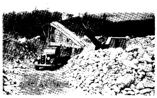
Power-shovel, loading-pocket, and truck, Inca Placer Pit, Palmer Bar Creek.
