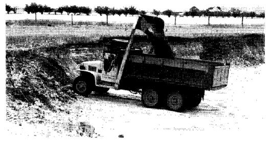
A. Dozer-loader attached to a 6-wheel drive General Motors truck, 7-yard capacity, excavating clay near Grand Forks.
