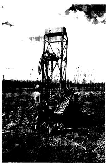
Drilling seismic holes in muskeg.
