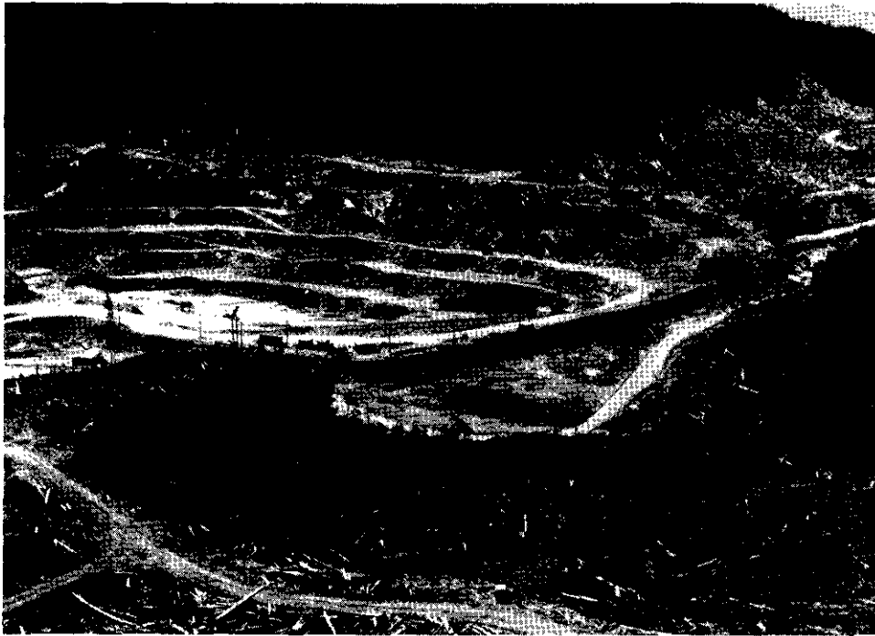
Brynnor Mines Limited open pit. Buildings are on dam built to divert Draw Creek from pit area.
