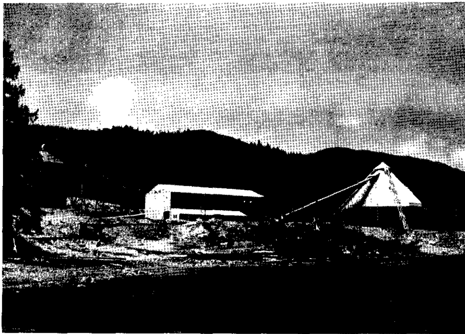
Brynnor Mines Limited. Fine-ore bin, mill, and concentrate stockpile on shore of Toquart Bay.
