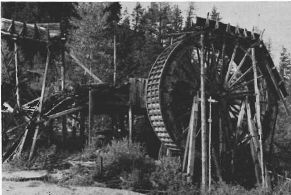
Overshot water-wheel on Perry Creek. This 32-foot wheel was built in 1933 and was moved bodily to Fort Steele in 1965 to form part of a historical exhibit.
