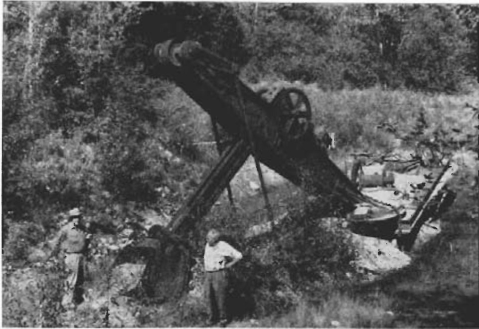
Old steam shovel on Perry Creek. This was a railway shovel, and it was taken in on sections of track under its own power in 1903.
