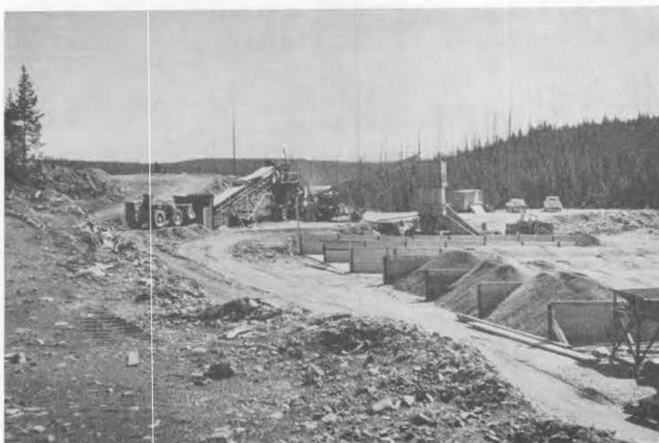
Brenda mine sampling operation showing the crusher and fine-ore bins, August, 1966.
