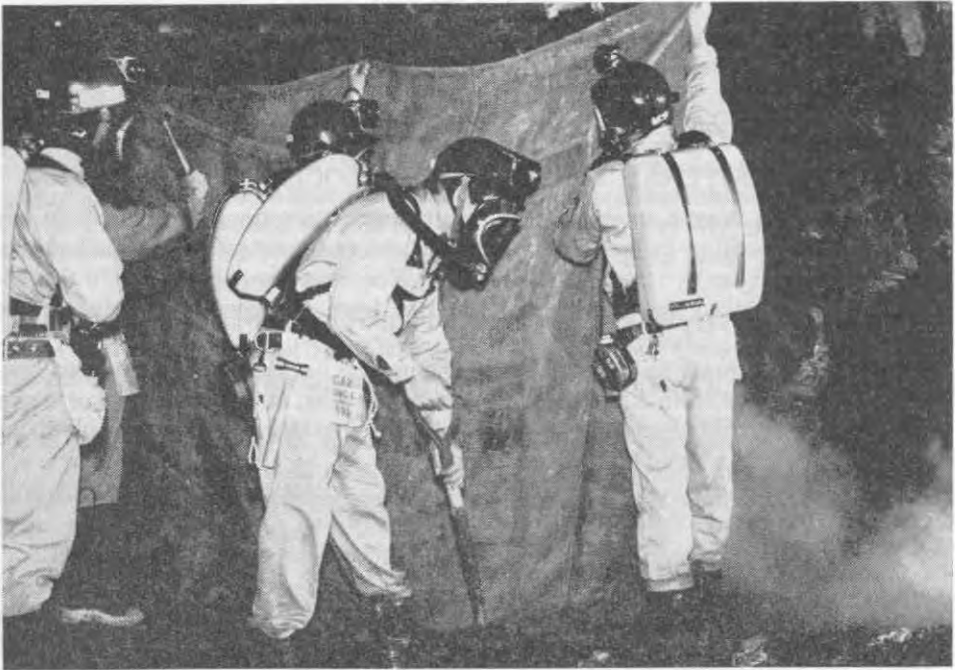
Mine-rescue team from Britannia mine erecting a fire seal underground.
