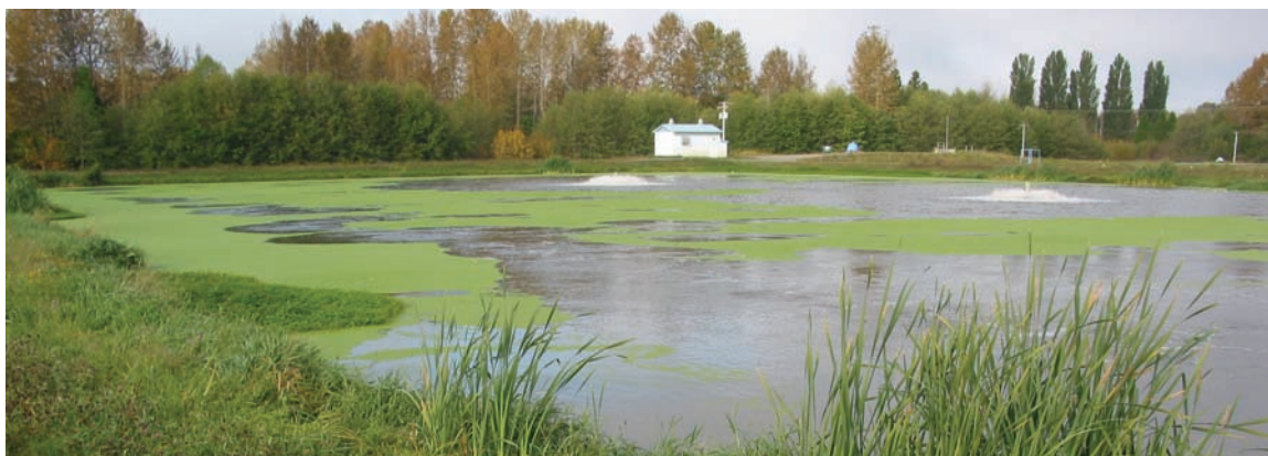
Figure 33. A secondary treatment lagoon at the Graham Avenue wastewater treatment plant, City of Terrace. Small fountains within the lagoon mix and circulate oxygen into the wastewater. This oxygen is essential to bacteria that feed on and digest the organic matter, converting it to non-harmful products. Abundant green algae and plants on the surface reflect the nutrient-rich nature of the wastewater. Photo by Bob Turner.
