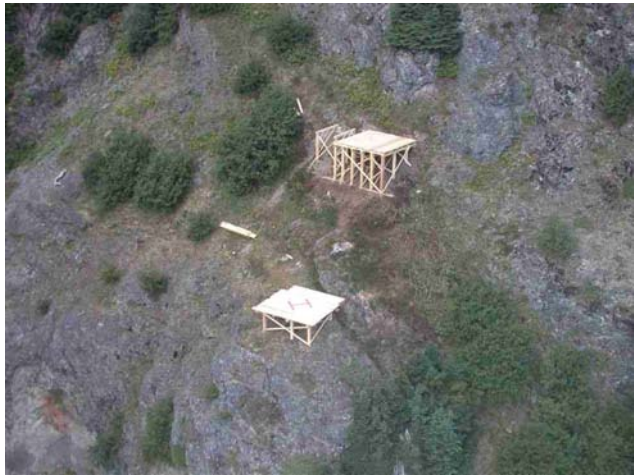
Photo 10. Drill platform under construction at the Rico gold vein showing on the Kalum property.
