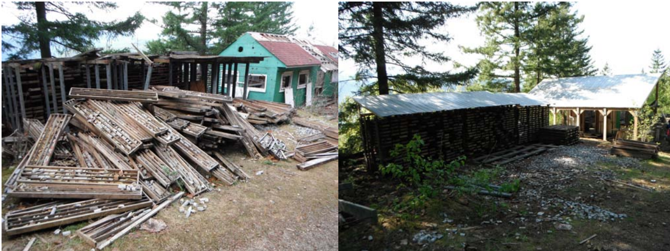
Figure 5.15. Before and after repair shots of the core storage and logging area at the Abo gold project. Vandalism and theft are intractable problems at accessible locations. This core was apparently dumped to gain access to the rebar used in the racks.
