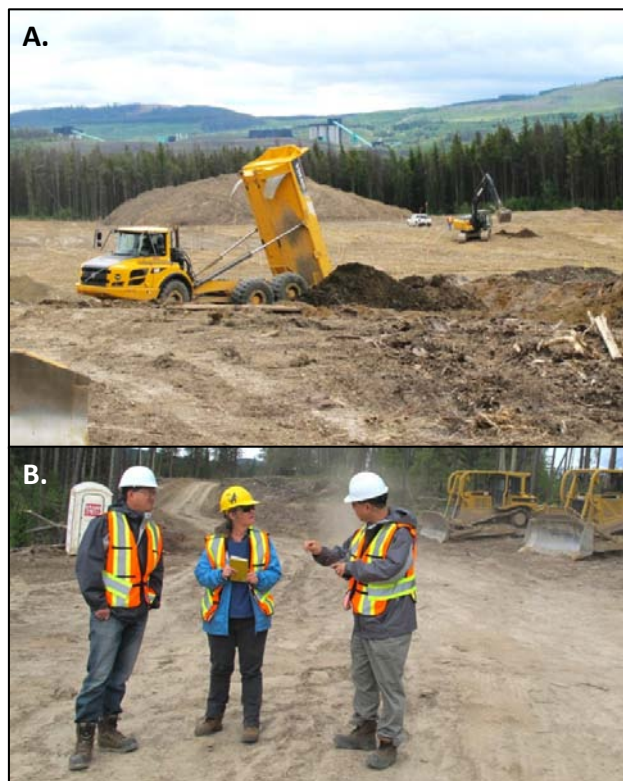
Figure 3.11. Murray River – A. Stripped and graded North Shaft site with soil stockpile and Quintette Mine in the background 3 km to the southeast; B. HD Mining Engineers discuss North Shaft site with Janet Riddell.
