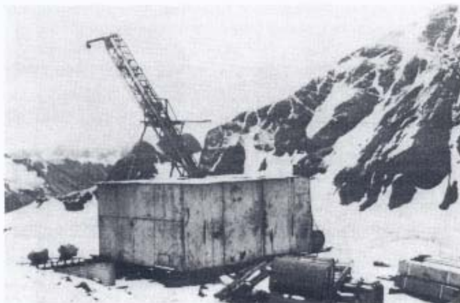
Photo 1. Summer diamond drilling at the Windy-Craggy copper-cobalt deposit. Indicated reserves 310 million tonnes at 1.50 per cent copper, 1 kilogram cobalt per tonne.
