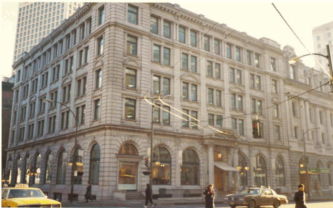
Fox Island granite – used in part to construct the Winch Building, Vancouver.
