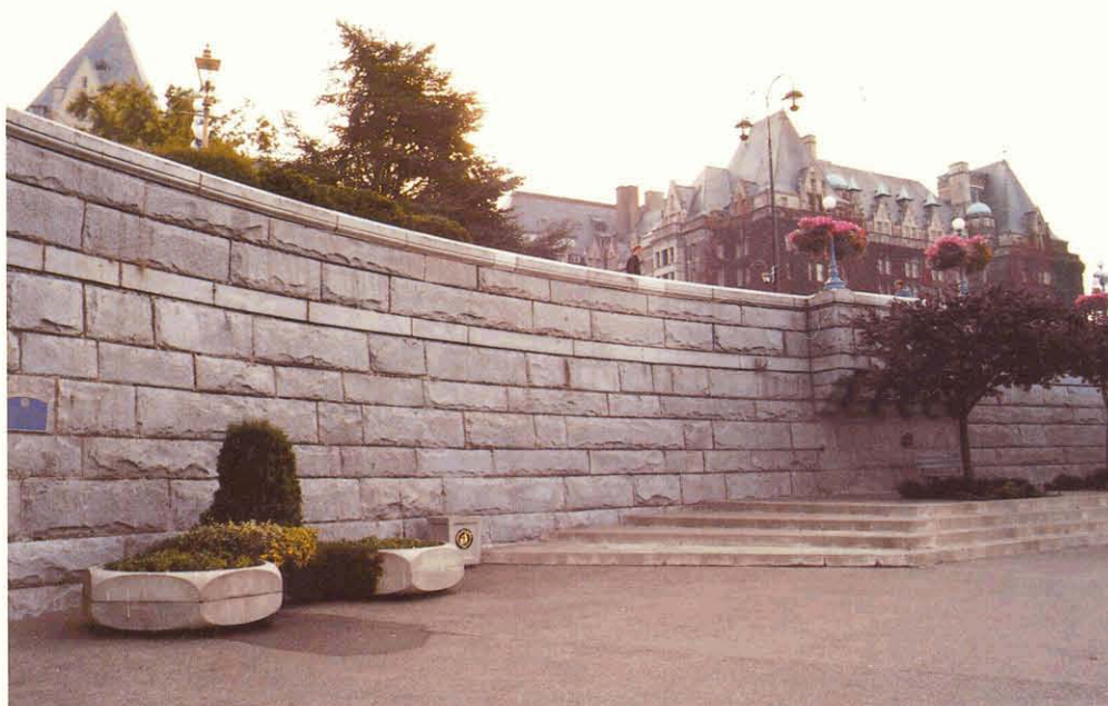
Kelly Island granite was used (in part) to construct this wall along the Inner Harbour, Victoria.
