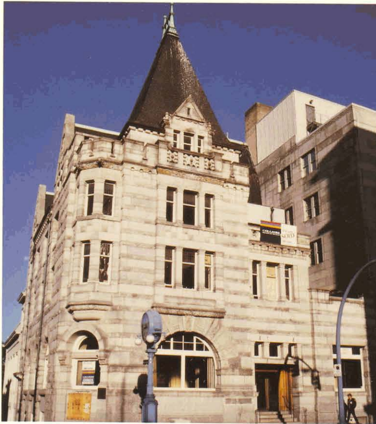
Haddington Island andesite – used to construct the Bank of Montreal, Victoria.
