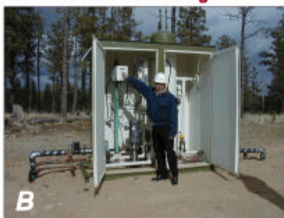
Gas- and water-metering station
