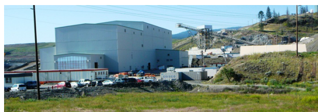
Photo 15. The ore conveyor emerges from the New Afton underground mine development scheduled for opening in 2012 after a five-leg, 4.5 km long journey from preparatory underground mining operations.
