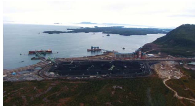
Photo 6. Expansion of the Ridley Island coal terminal near Prince Rupert is underway and receives fill material from nearby quarries. Increased coal shipments through this port from a variety of coal fields are anticipated.
