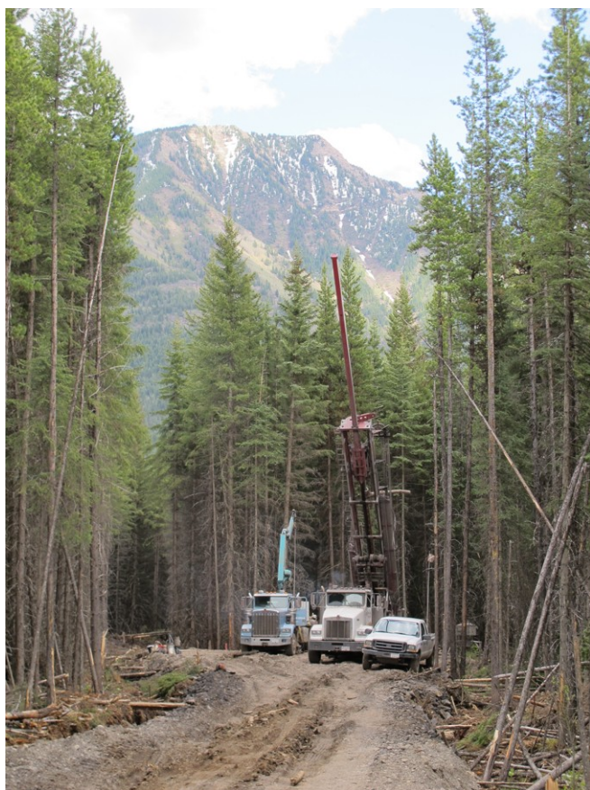
Figure 6: Geotechnical exploration drilling on the Bingay Creek coal property of Centermount Coal Limited.
