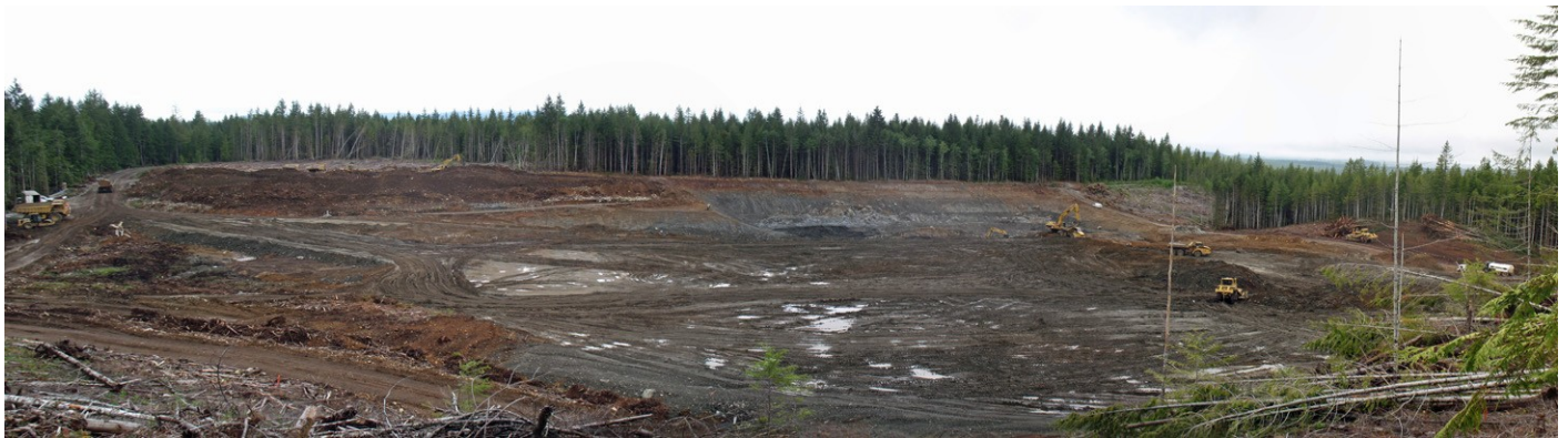
Figure 5: Site preparation of the 7 South area at Quinsam Mine, Vancouver Island. A coal seam is exposed in the centre of the frame.
