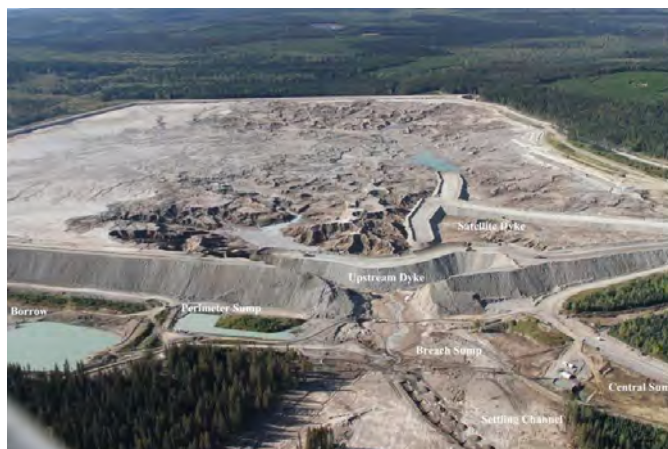
Fig. 6. Repairing the breached tailings dam at Mount Polley mine, September 2014. Photo courtesy of Imperial Metals Corporation.
