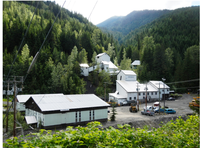
Fig. 18. Klondike Silver Corp's (Slocan Silver) mill at Sandon.
