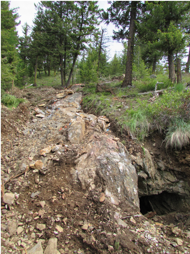
Fig. 19. Trenching at the Gold Drop-North Star vein system, near one of the historic adits on the property.
