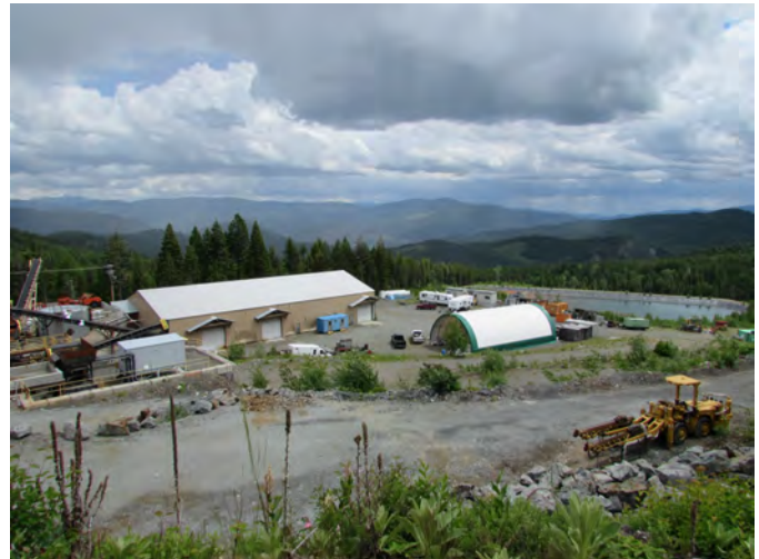
Fig. 13. The 200 ton-per-day Lexington mill (gravity-flotation) and tailings facility. Golden Dawn Minerals Inc. has entered into a purchase agreement with Huakan International Mining Inc. to acquire both the Lexington mine and mill, as well as the nearby Golden Crown mine. Both mines are underground Cu-Au mines.
