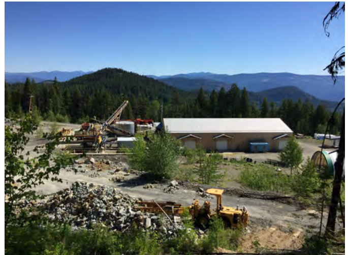
Fig. 12. The 200 tpd Lexington mill (gravity-flotation) and tailings facility.
