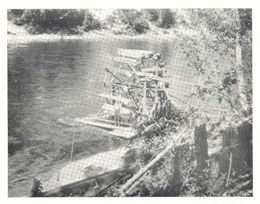
A Current-wheel on the Nechzko River. The wheel is 16 feet in diameter with a 9-foot face. Note the buckets for raising the water on the near side of the wheel.
