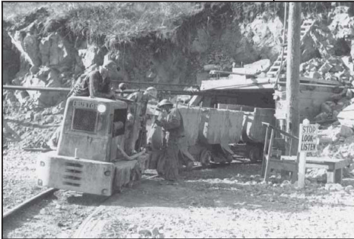
Photo D18. Portal of the HB lead-zinc mine developed mainly by adits. The photo shows one of the first diesel locomotives used underground emerging from the 2800 level. (Matt Hedley, AR 1956)
