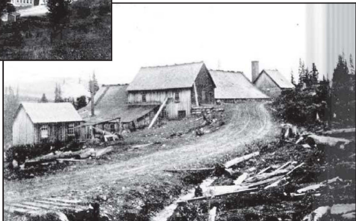
Photo D8. The provincial government's reduction works near Barkerville in 1902. This first primitive test mill and smelter was built in 1888 to stimulate exploration and mining of pyritic gold-quartz veins in the district as placer production decreased. The technology of the day was unable to adequately release the gold from the pyrite. (AR 1902)
