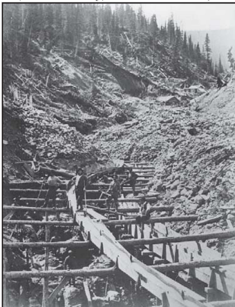
Photo D3. A placer mine on Williams Creek in 1867 that, unlike most of that time, exposes the workings to view rather than being underground. Note the central flume and sluice box, miners shoveling in gravel at the upper end and cleaning up bedrock in the foreground, and the stacked boulders - an eternal problem. (Fredrick Dally, BCARS HP 94703)
