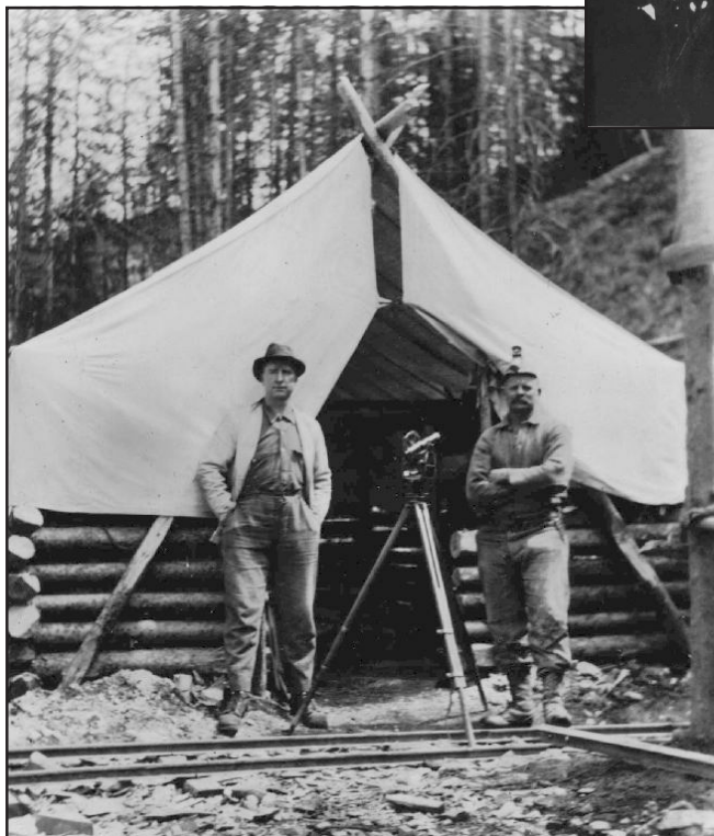
Photo A5. Early surveys of prospects by the Bureau or Mineral Survey were conducted by pace and compass or, less commonly, by transit and chain as shown here at the portal of the Revenge mine at Beaverdell in 1921. Reconnaissance surveys were only crudely controlled geographically. (BCARS HP 99682)
