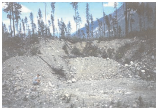
Figure 3. Typical borrow pit used to facilitate logging road construction. Pits are generally small ( \sim 2000\text{m}^3 ) and exploit local material to reduce transportation distance (forest service road south of Birkenhead Lake).
