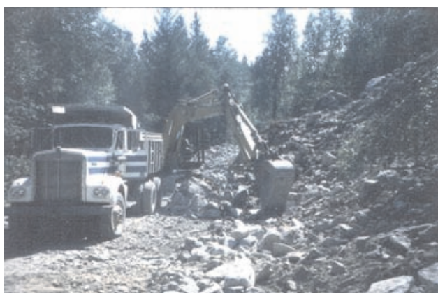
Photo 2. Active mining of the colluvium along Lillooet Forest Service Road, in the upper Lillooet River Valley. Material here is being used to armor river banks (rip-rap) along reaches where erosion threatens the logging road. Other locations provide aggregate for road base and diking material.
