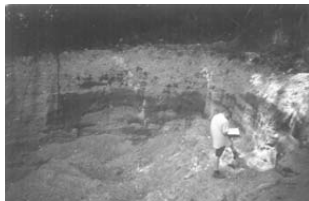
Photo 1. An example of a small borrow pit located near the town of Gibsons where material is being extracted for road construction on private land.
