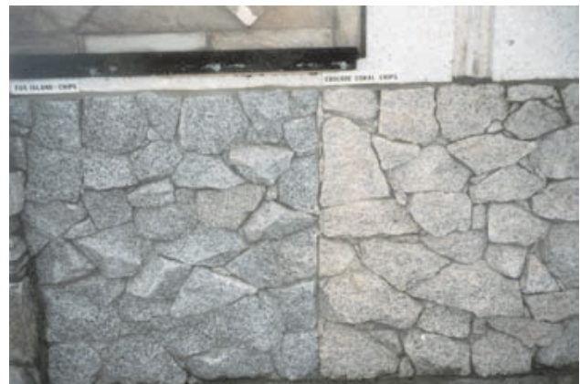
Photo 12. Typical use of stone chips (rubble) in wall facing. BC granites from Fox Island (left) and Beaverdell (right). Quadra Stone Company Ltd. product.
