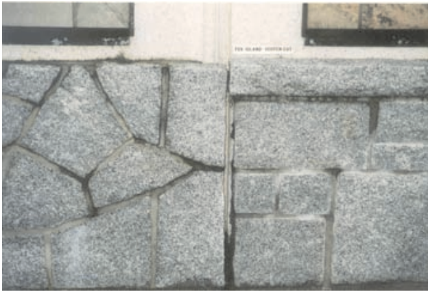
Photo 10. Typical use of split stone in wall facing. BC granite from Fox Island. Quadra Stone Company Ltd. product.
