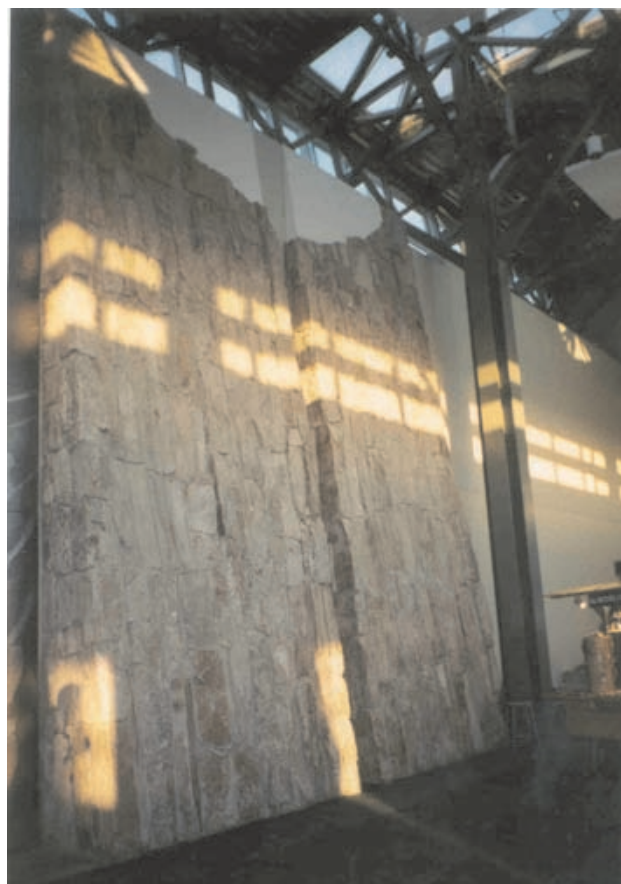
Photo 14. Split columnar basalt from Whistler as a wall facing, Vancouver airport building. Garibaldi Group product.
