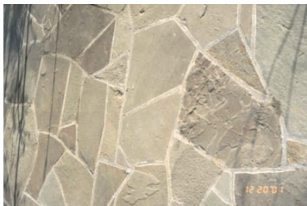
Photo 8. Bowen Island home patio floor. Cut, irregular shape slabs of 1 to 2 square feet (900 to 1800 square centimeters) in size.
