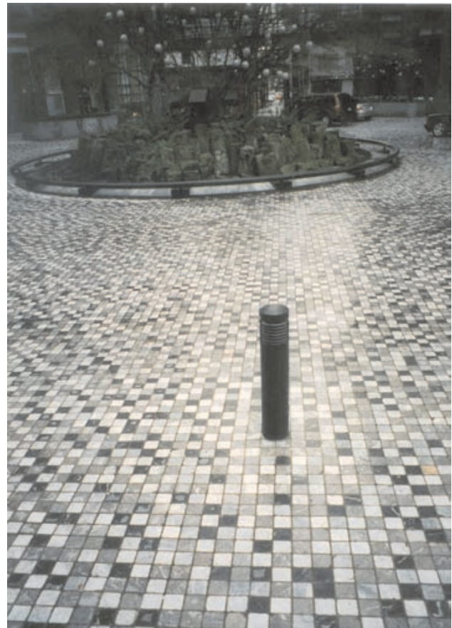
Photo 11. Vancouver Island marble varieties. Mosaic floor assembled of 10 by 10 centimetres square cut pavers (tiles). Matrix Marble Corporation product.
