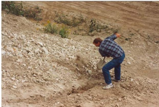
Figure 5. Exposing the bedrock for channel sampling.
