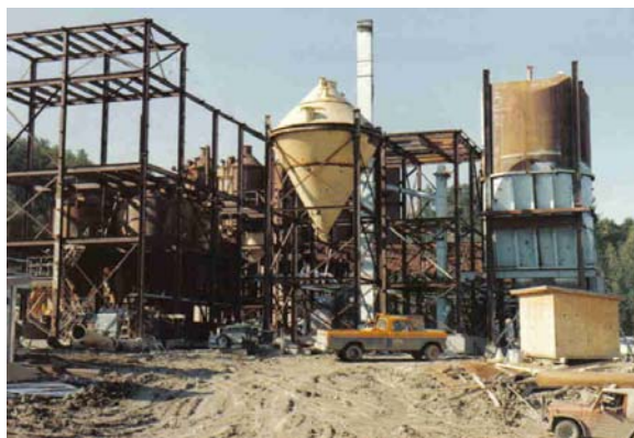
Figure 39: Microsill plant (1982 photo). The diatomite rock from the Crownite deposit was calcined and transformed into a variety of absorbent products. Photo used with permission of Mr. Garry Miller, one of the contractors involved in the design and construction of this plant.
