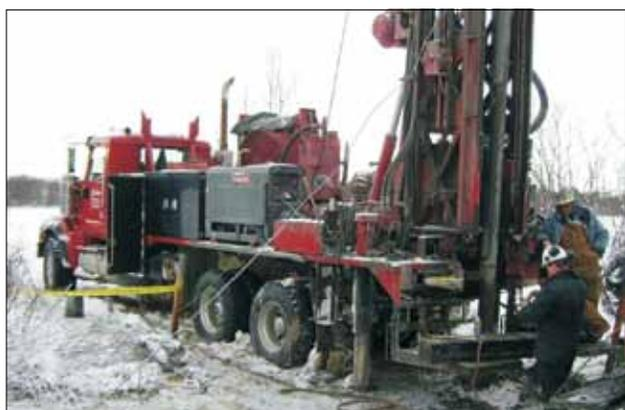
Figure 5. In November 2011, six new water observation wells were drilled along on road rights-of-way using an air rotary water well drilling rig with a casing hammer.
