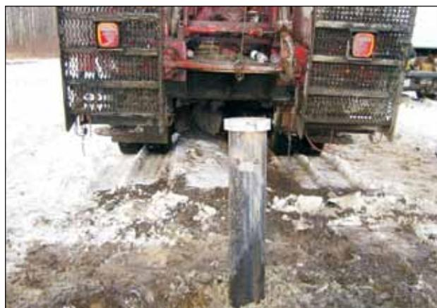
Figure 6. Following completion, approximately 1.5 m of steel casing remained above ground to mark the well. The casing was tagged with a well number and a lock cap was installed.
